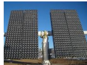
CPV power system
